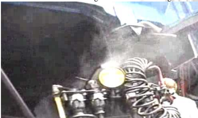
Detailed view of excessive smoke in a motor running
