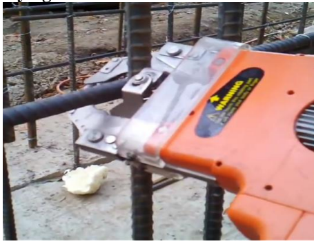
Figure 4: Rebar tying machine
