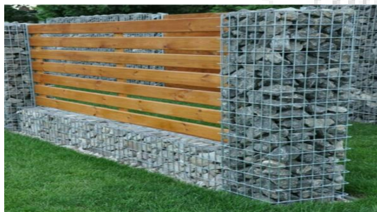
Figure 10: Gabion walls
