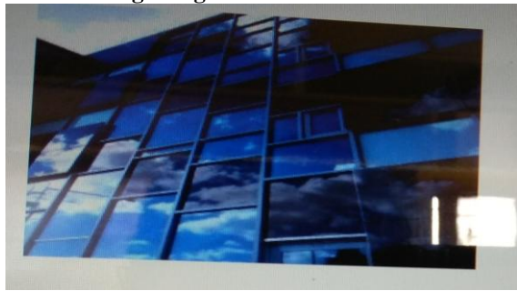
Figure 8: Photovoltaic glazing
