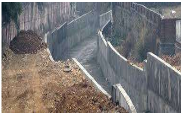
Figure 9(b): Photograph of a RCC drain
