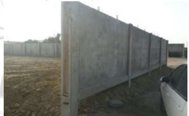
Figure 8(b). Photograph of a RCC Retaining wall
