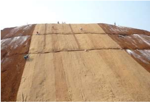
Figure 7(a). Jute Geotextile for Erosion Control
