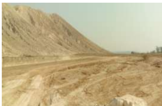
Figure 3: Deep rain cuts in OB dump
