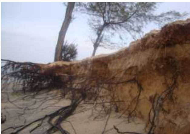
Plate 1: A severe wave action observed along the coast due to the sudden change of beach profile as steeper
