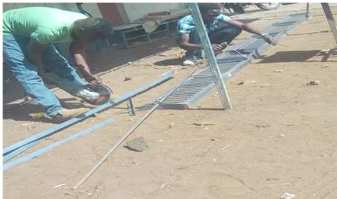
Plate 1: Iron workers without PPE and in bending/stooping posture
