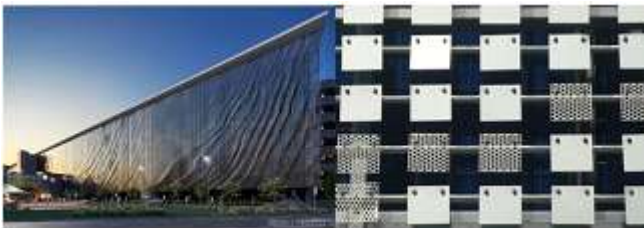
Figure 13: The kinetic wall of Brisbane airport garage and its panels [25]
