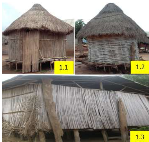
Plate 1: "Ago" at Tan-Adja and at Agongbodji
