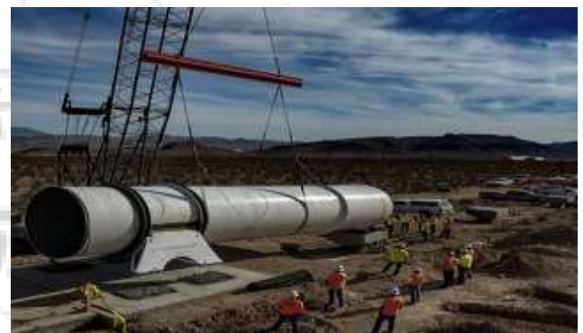
Figure 2: Construction of tube
