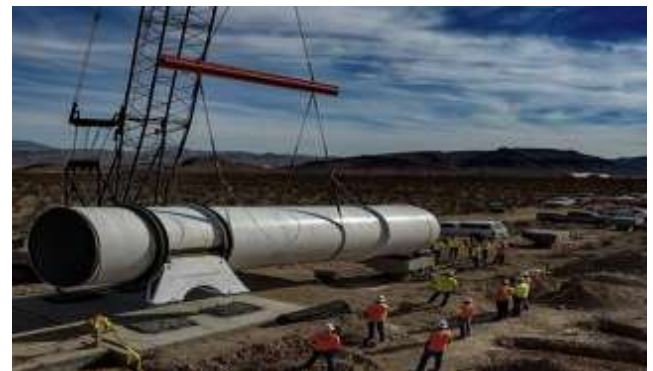
Figure 2: Construction of tube
