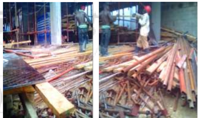
Plate 4.01: (Left) worker working on a site with untidy hazardous materials; and (Right) hazardous steel material stored untidy within the site, Source: Author,(2017).
