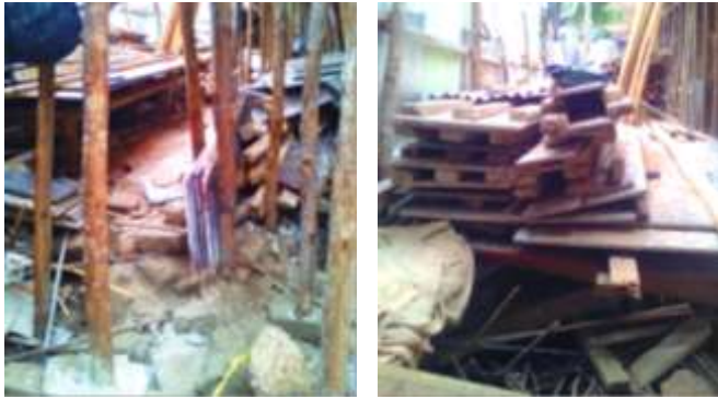
Plate 4.02: (Left) hazardous wooden materials stored untidy within the site; and (Right) hazardous waste materials stored untidy within the site, Source: Author,(2017).
