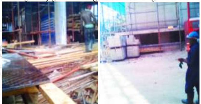
Plate 4.06: (Left) lack of protective clothing hazard; and (Right) a worker with protective clothing, Source: Author,(2017)
