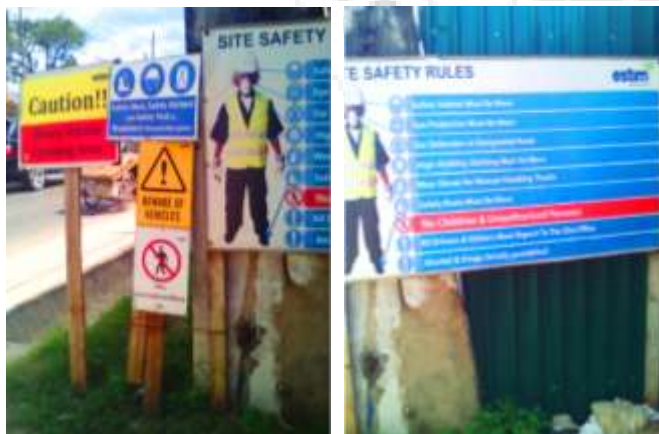
Plate 4.09: (Left) safety policies outside site compound; and (Right) safety rules within the confined site, Source: Author,(2017).
