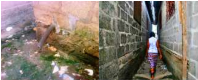
Figure 4.02: (Left) a photo of a pit latrine showing the emptying pipe at the base; and (Right) the main access road and some of the narrow foot paths used to access the slum areas
