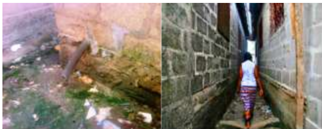
Figure 4.02: (Left) a photo of a pit latrine showing the emptying pipe at the base; and (Right) the main access road and some of the narrow foot paths used to access the slum areas
