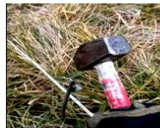
Driving stakes into the ground using 5 lb. hammer
