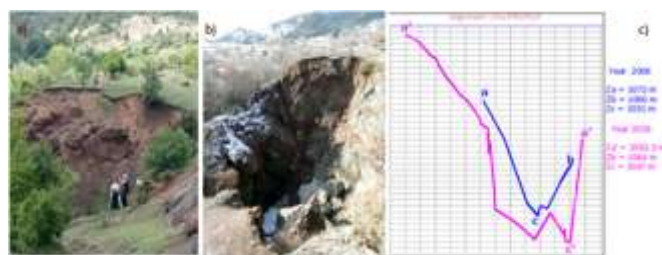
Figure 2: Environmental damage at Rehova copper mine. (a) Survey of a sinkhole. (b) Image from the sinkhole. (c) Presentation of the size of the funnel in a cross section, the sinkhole size in 2006 (blue line) and in 2018 (magenta line)
