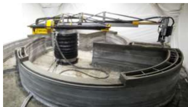
Figure 1: An ApisCor mobile 3D printer printing a concrete structure
