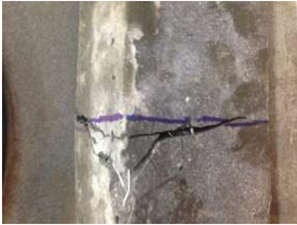
Figure 10: Mode of failure in reactive powder concrete hook end steel fiber for prism.
