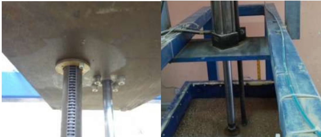
Figure 3: Steel plate to support the hydraulic jack
