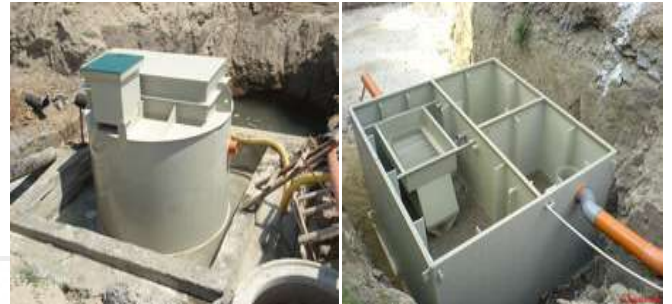
Figure 18: Concept WWTP for Home Based Enterprise (HBE)
