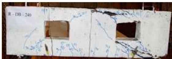
Figure 10: Crack pattern at ultimate load for beam R-DB-240 (Group A) (shear – compression failure)
