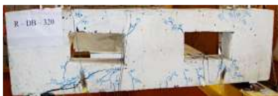
Figure 11: Crack pattern at ultimate load for beam R-DB-320 (Group A) (diagonal splitting failure)
