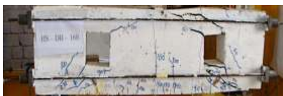
Figure 12: Crack pattern at ultimate load for beam HS-DB-160 (Group B) (diagonal splitting failure)
