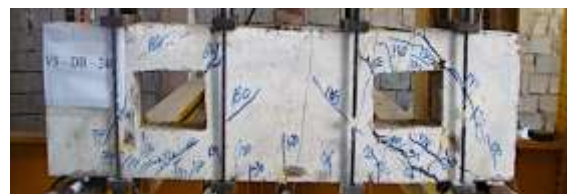
Figure 16: Crack pattern at ultimate load for beam VS-DB-240 (Group C) (shear – compression failure)
