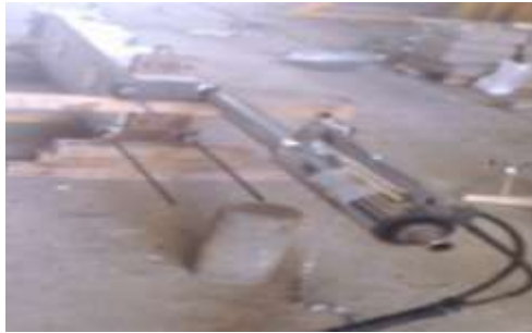
(a) Jacking stress process for beams with horizontal strengthening strands
