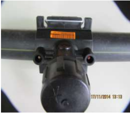
Figure 6: Elbow - polyethylene pipe Dn63-32 assembly resulting from electro-fusion welding
