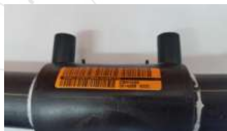
Figure 1: Pipe and fitting following the polyethylene welding
