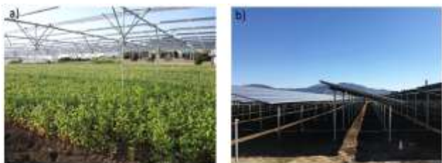
Figure 1: a) Project A: small-scale 50 kW agro-photovoltaic project, b) Project B: large-scale 20 MW agro-photovoltaic project, in Tsukuba, Japan. Note that the picture b) is taken shortly after finishing construction; therefore no agricultural activity is yet visible
