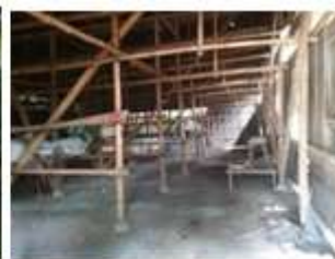
Source: Survey, 2016 Figure 13: Space in tobacco warehouse
