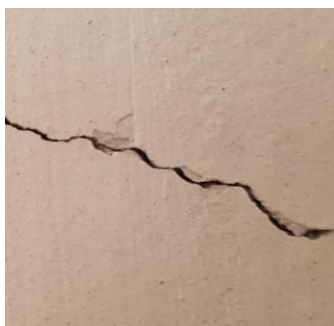
Figure 1.1: Crack on a surface wall
