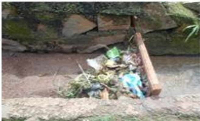
Figure 4: Waste captured by soil trap after a rain event
