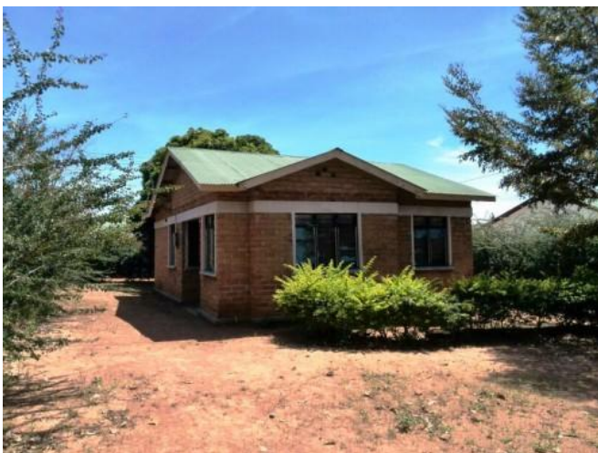
Figure 2: A clay burnt brick house in Iringa town
