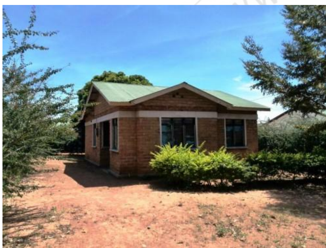
Figure 2: A clay burnt brick house in Iringa town
