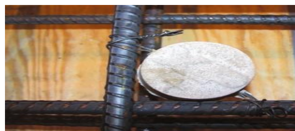
Figure 9: Installation of an embedded sacrificial anode.
