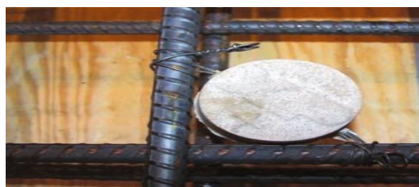
Figure 9: Installation of an embedded sacrificial anode.
