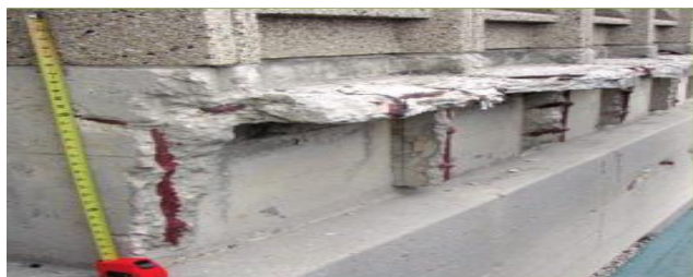
Figure 3: Spalls in concrete
