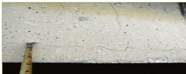
Figure 2: Cracks in Concrete
