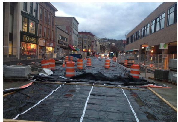
Figure 6.1: Curing Process in Extreme Weather
