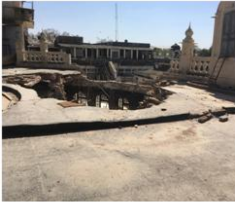
Figure 1: Roof of commissioner hall
