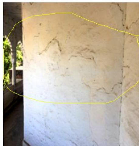
Figure 2: Wall of labour court Width- 1mm Type- Medium (Non-structural crack)
