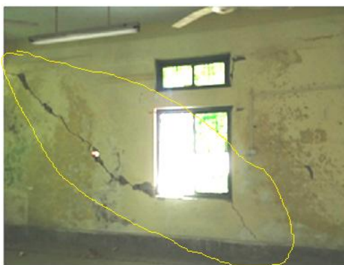
Figure 2: Long Wall of Sir Alexander Cunningham hall (political block) Width- above 2mm Type- Wide (Non-structural crack) Shape- Stair step crack Cause- settlement of foundation.
