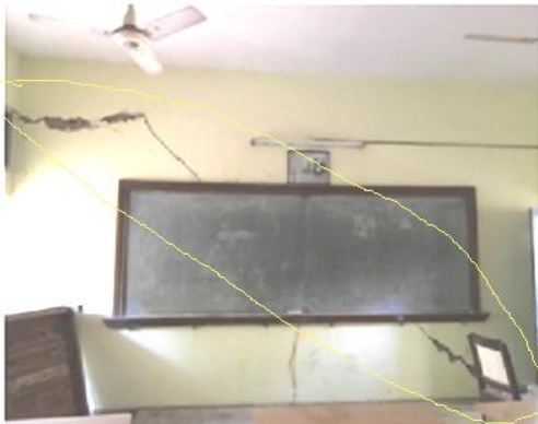
Figure 1: Short wall of classroom 16 (political block) Width- above 2mm Type- Wide (Non-structure) Shape- Diagonal, Horizontal crack Cause- settlement of foundation
