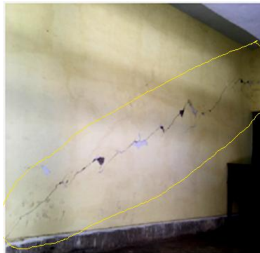
Figure 4: Wall in archaeological block Width- 1 to 2 mm Type- medium, non-structural crack Shape- diagonal Cause- settlement of foundation
