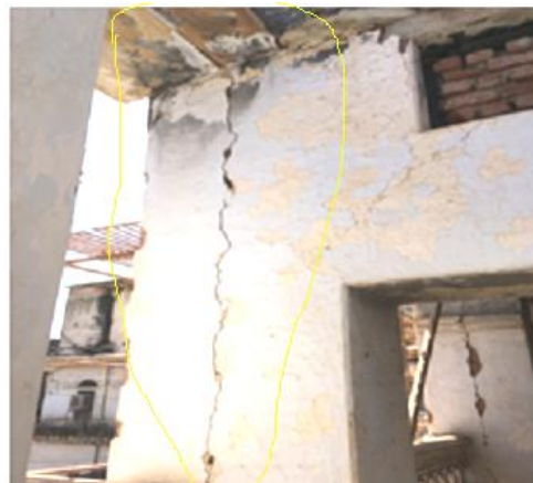
Figure 1: Column at industrial court Width- 2mm Type- Major structure Crack Shape- vertical crack Cause-thermal variation, due to joint
