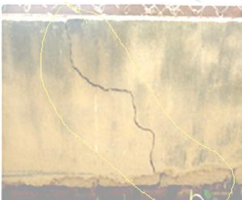
Figure 1: Exterior wall of hostel building
