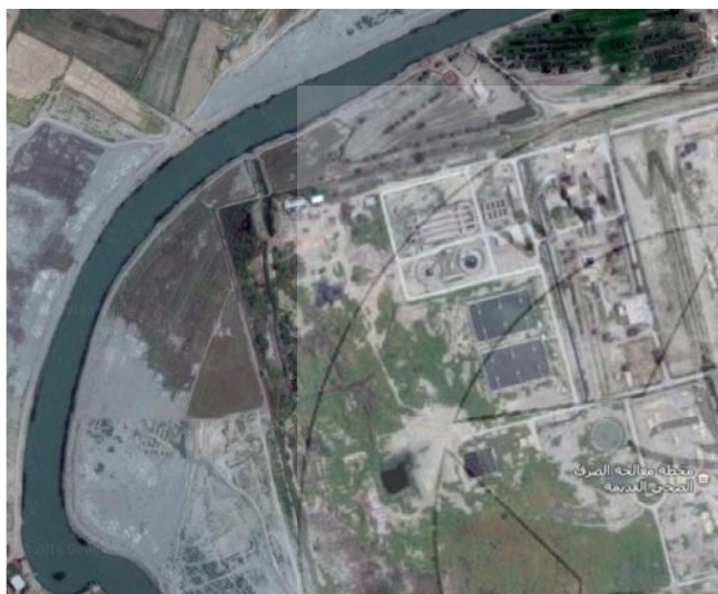
Figure 1: Al-Diwaniyah WWTP site location
