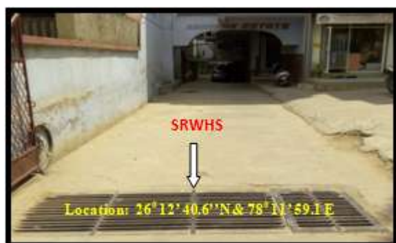
Figure 9: Surface rain water harvesting structure
