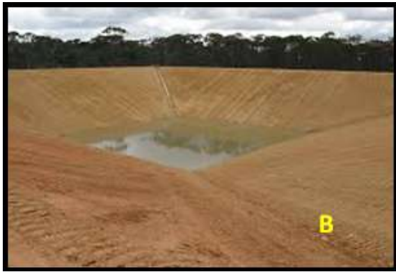
Figure 4 B: Recharging pit
