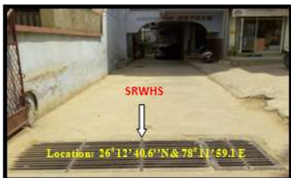
Figure 9: Surface rain water harvesting structure
