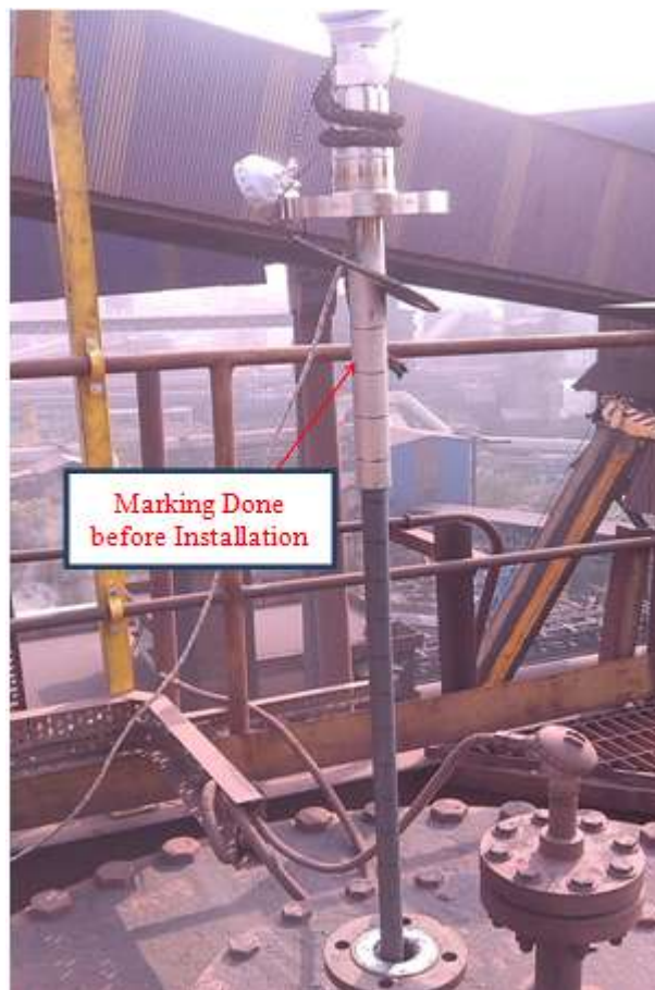
Figure 7: Installation of Dome Thermocouple at I Blast Furnace, Tata Steel Jamshedpur.
