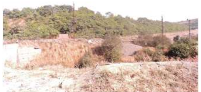
Figure 8: Plantation on the top of the dump.
