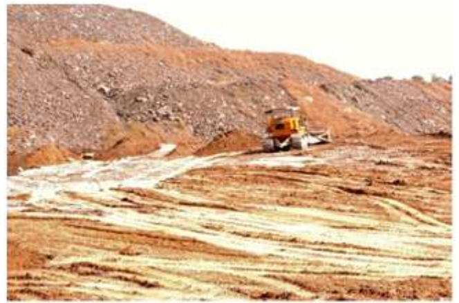
Figure 7: Spreading and compacting admixture of fly ash and overburden
