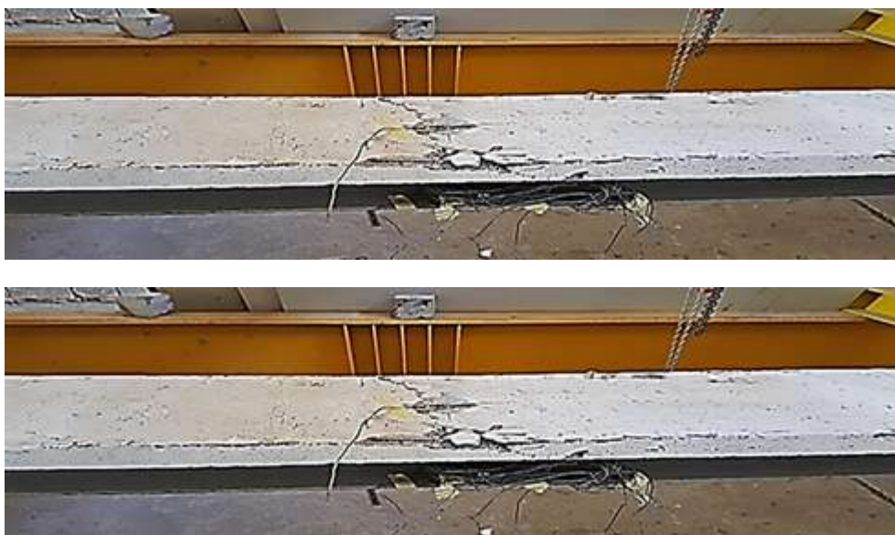
Figure 6: The Mode of Failure of the Steel Girder (GP9S-e80) G1
