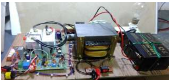
Figure 3: Photograph for the prototype of the designed bidirectional inverter
