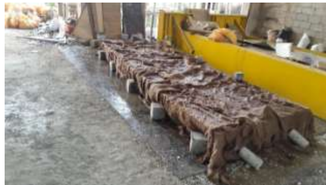
Figure 5: final stage of construction (Model BGC R 23.3)
