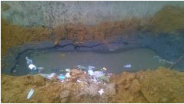
Figure 10: Hole dug to accommodate the products of a manual draining in Avocatier-Agnissankoi
