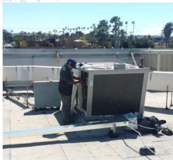
Figure 5.1: Installation and maintenance of ice bear unit
