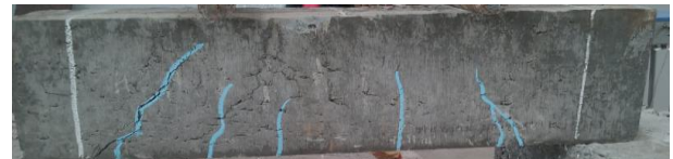
Figure 10: Crack pattern of control beam
