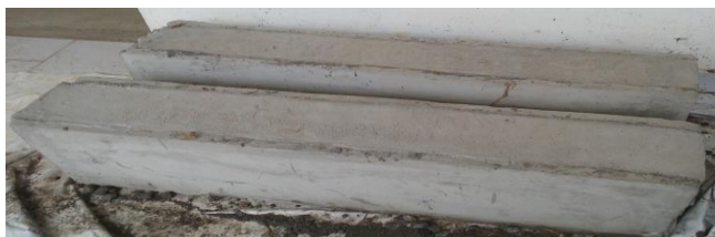
Figure 5: Beam with ferrocement formwork after casting
