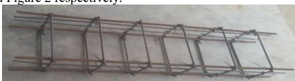
Figure 1: Reinforcement for control beams
