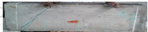
Figure 11: Crack pattern of beam with ferrocement formwork having single layers of chicken mesh
