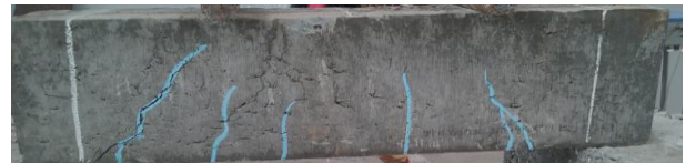
Figure 10: Crack pattern of control beam
