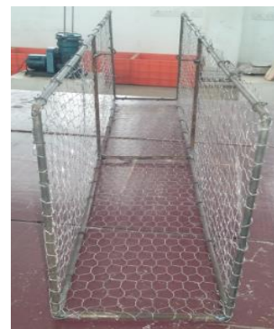
Figure 3: Skeletal reinforcement covered with chicken mesh
