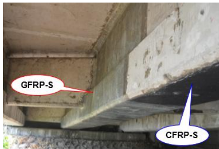
Figure 3: Application of CFRPs and GFRPs on Malelleng's Bridge
