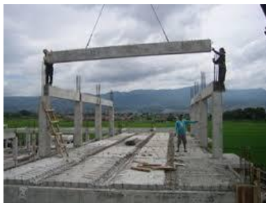
Figure 1: Assembling of precast members
