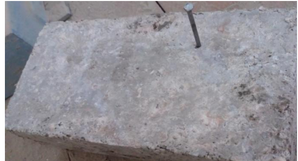
Figure 3.6.1: Nail in the brick
