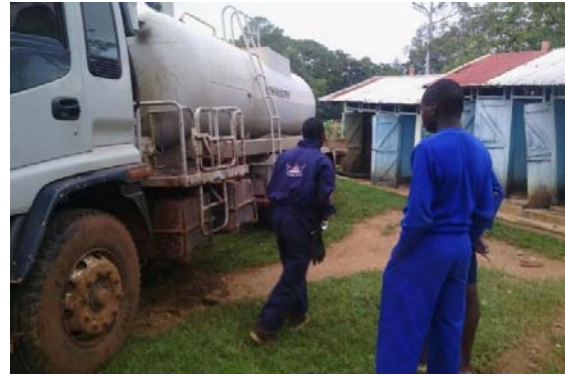
Plate 2: Mechanical means of emptying pit latrines
