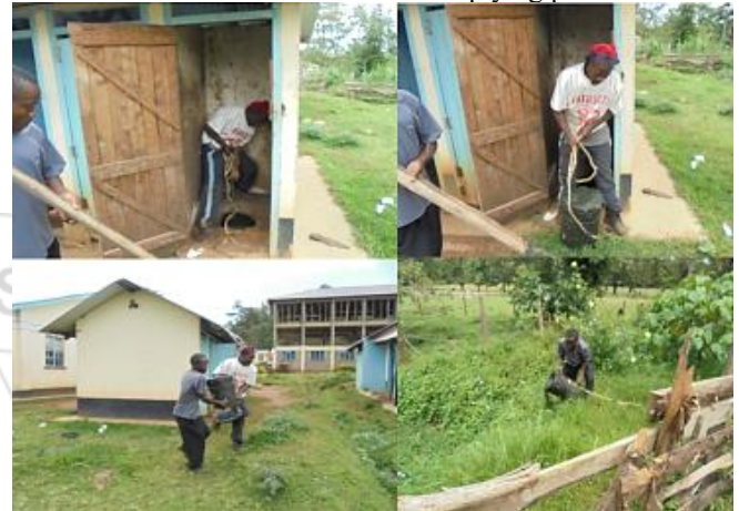
Plate 3: Manual means of emptying pit latrines
