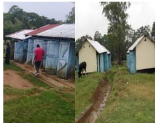
Plate 1: Common human waste disposal systems in schools
