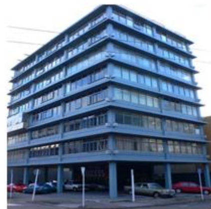
Figure 1: Building with ground floor as soft storey
