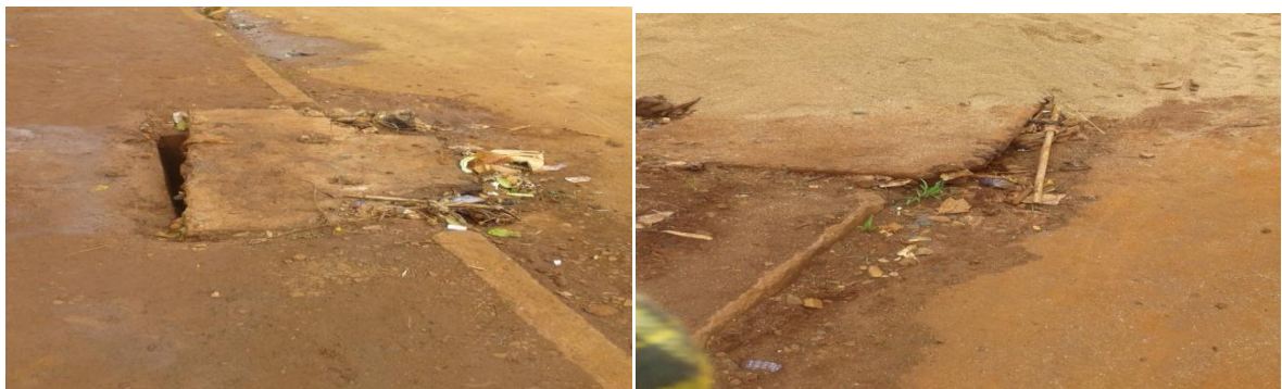
Figure 5: Poorly Executed Manholes
