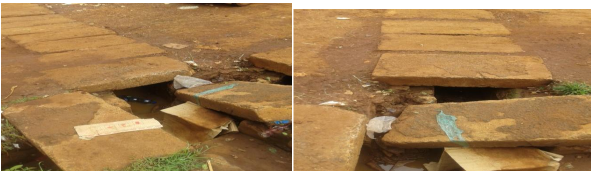
Figure 6: Poorly Covered open drains
