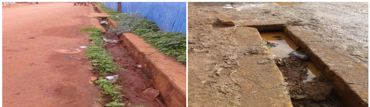
Figure 4: Failed & blocked Side drains
