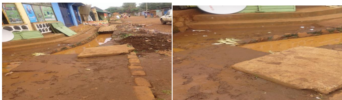
Figure 2: Rectangular Open Drains with poorly defined outlet
