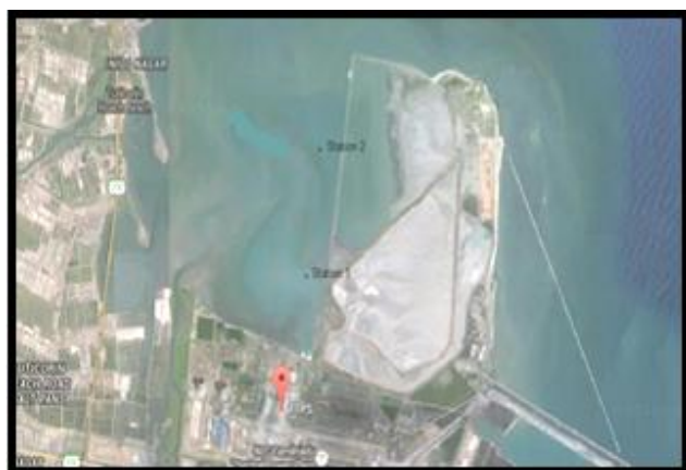
Figure 1: Aerial view of Tuticorin Thermal Power Plant (TTPS) with 2 stations
