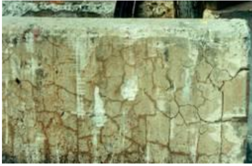
Figure 4: Alkali silica attack
