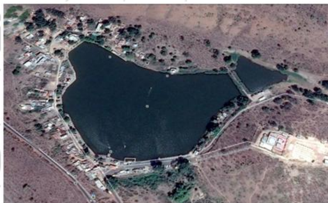
Figure 1: Image of Ambala Water Tank, Ambala, Ramtek (Source: www.googleearth.com , image collected on dtd September 15, 2014)
