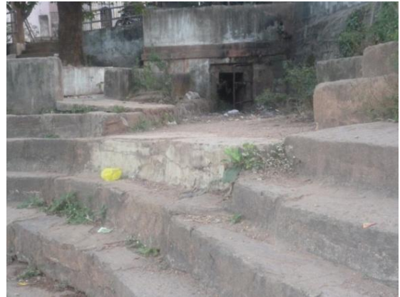
Figure 10: Drains opening into the Ambala tank (Photo Courtesy: the Author)
