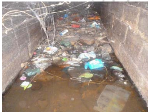
Figure 9: Solid Waste along with the plastic bags thrown into the drains leading to Ambala tank (Photo Courtesy: the Author)
