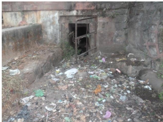
Figure 9: Solid Waste thrown into the drains leading to Ambala tank (Photo Courtesy: the Author)
