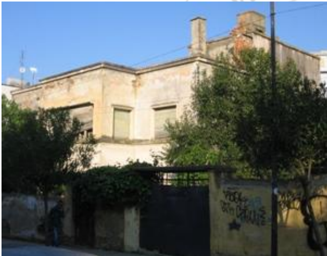
Figure 7: b) Building N°3 [8]
