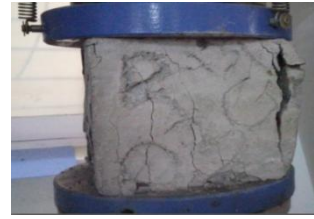
Figure 6: Compressive testing of cubes
