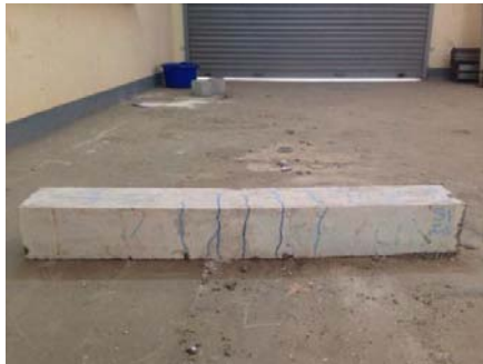
Figure 17: Crack pattern of S1CS specimen
