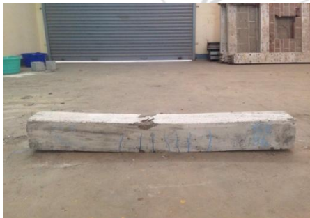
Figure 19: Crack pattern of S3SL specimen
