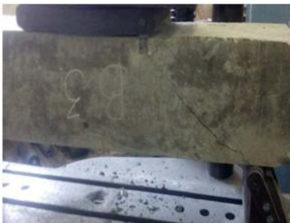
Figure 3: Diagonal Crack in Reinforced Beam
