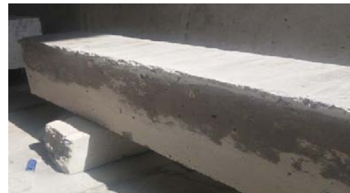
Figure 3: Concrete surface smoothing
