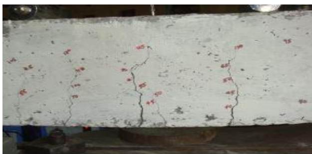
Figure 7: Flexural failure in control beam
