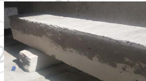
Figure 3: Concrete surface smoothing
