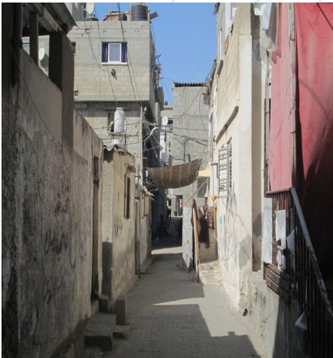
Figure 4: Jabalia camp poor roof materials, Source authors, 2016
