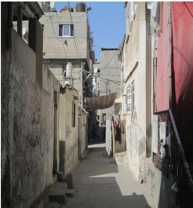
Figure 4: Jabalia camp poor roof materials, Source authors, 2016
